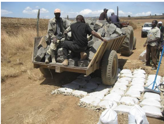
Figure 6. “Do-nou” bears the load of a heavy tractor during construction (Kenya)
