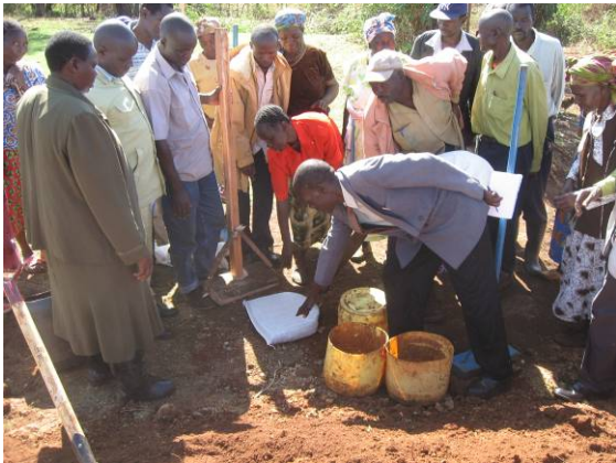
Figure 5. Kenyan farmers assessing the hardness of “Do-nou” after compaction.
